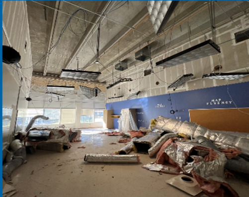
Ceilings and Ductwork Removed in Classrooms
