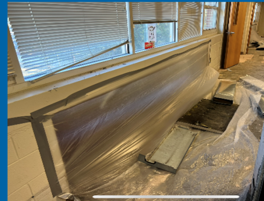
HVAC Equipment Removed from Classrooms
