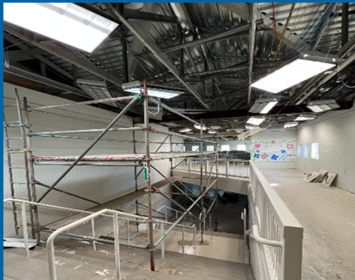
Ceiling and Ductwork Removed in the Gym Area
