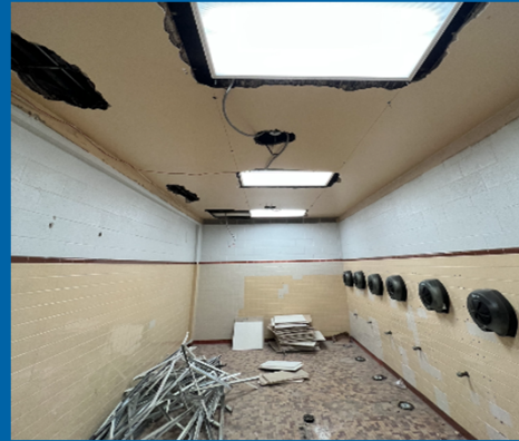
Toilets, Sinks, Partitions, and Ceilings Removed from the Bathrooms
